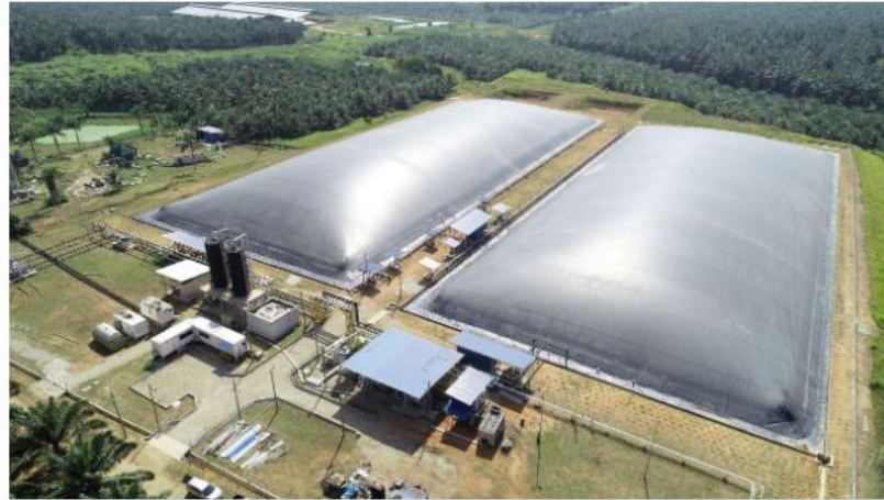
Aerial view of Johor Plantations' biomethane plant
