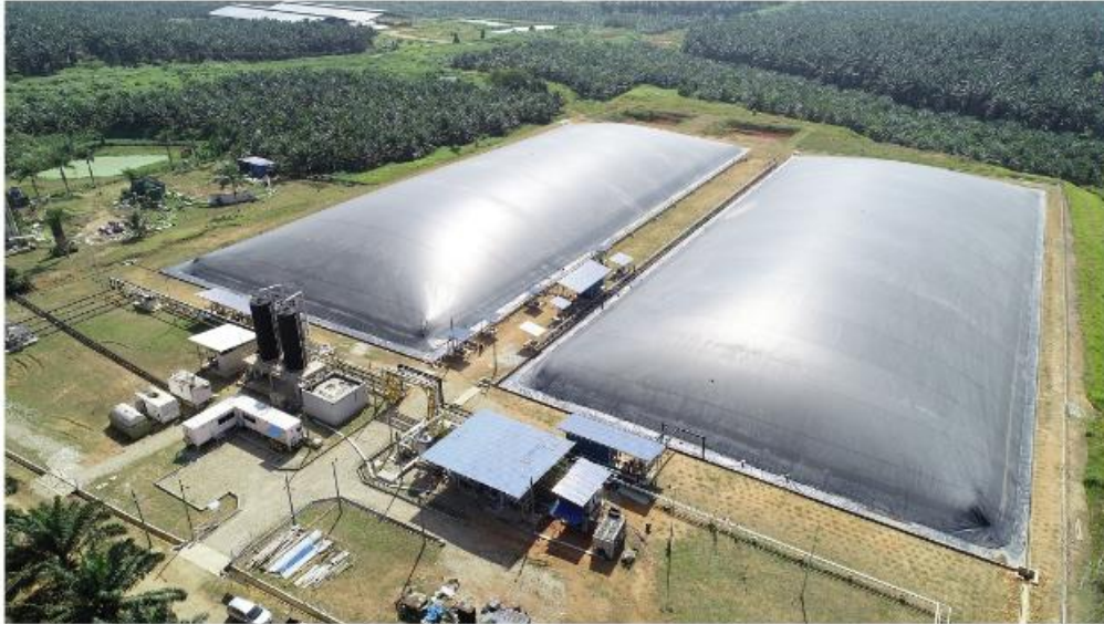
Aerial view of Johor Plantations' Biomethane Plant in Sedenak, Johor.
